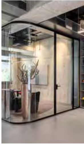
A very elegant detail is the round corner solution of the single office.
