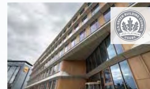
Project: ENTEGA AG, Darmstadt Certificate: LEED Platin
